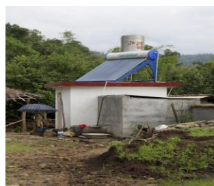
The best toilet facility (not requiring inclusion in the project) with a solar-powered water heater on the roof.
