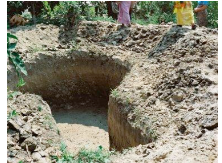
Toilet upgrade under construction
