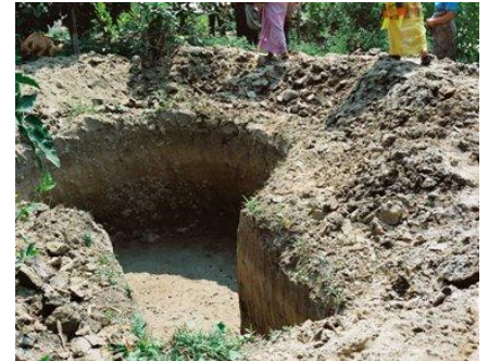
Toilet upgrade under construction
